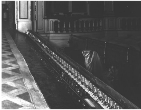
Adelphi Theatre - microphones seen across the front of the stage in front of the foot lights.
