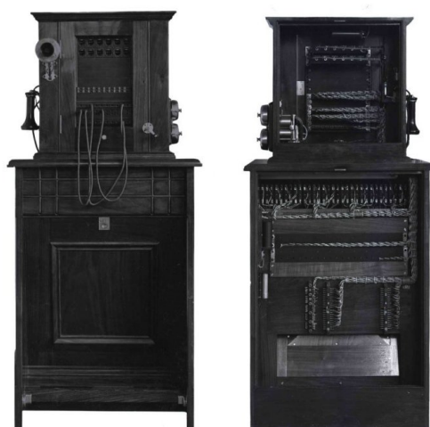
Electrophone Switchboard - Front and rear (Picture taken 1907)
